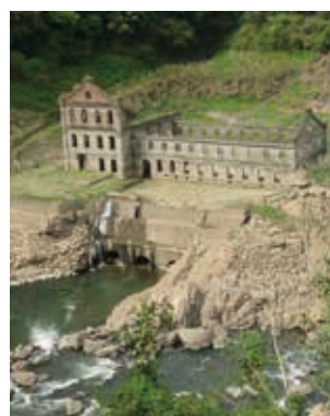
Ruins of the Old Hydropower Station (Sogi Electric Company)
